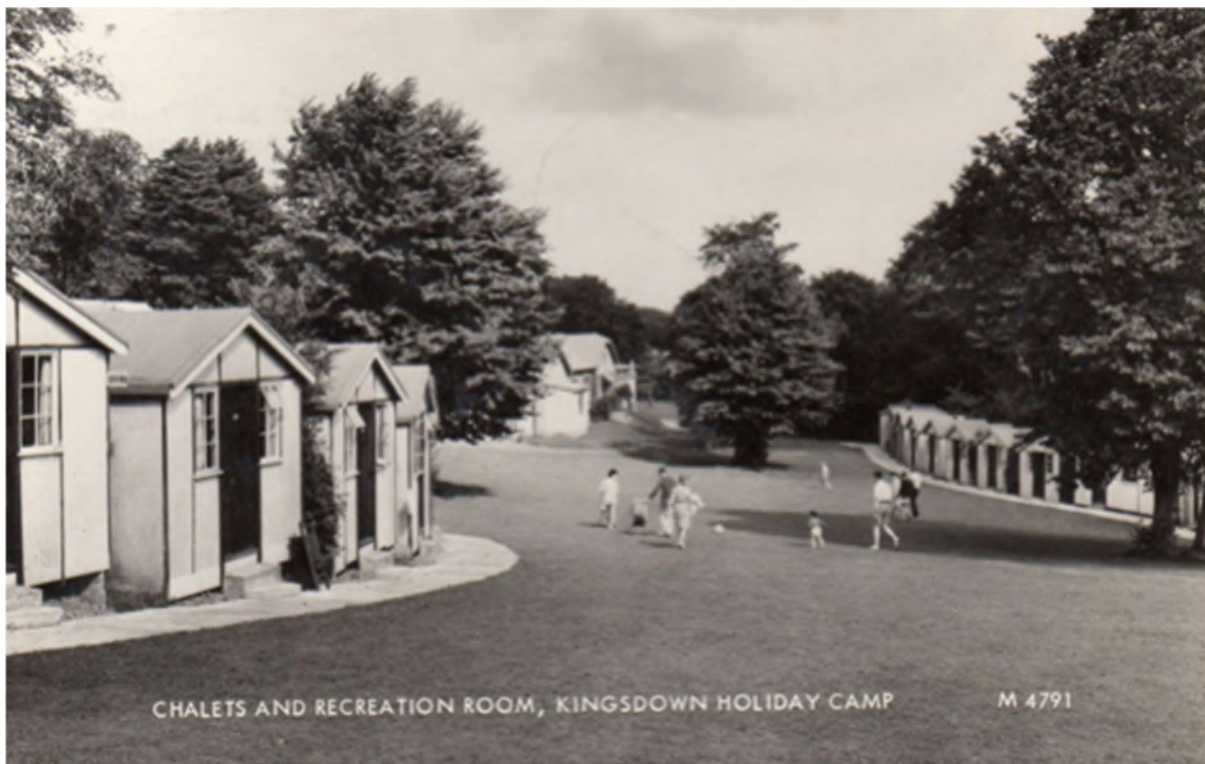
Figure 3 - Chalets and Recreational Room Kingsdown Holiday Camp
